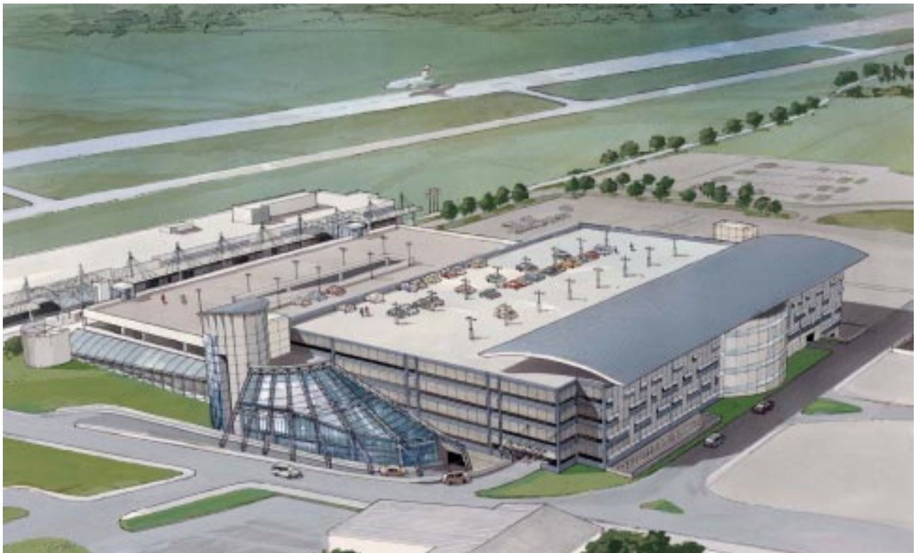
Top photo: The Jetport's General Aviation area with the new parking garage construction underway. Bottom photo: Artist Rendering of the new parking garage.
